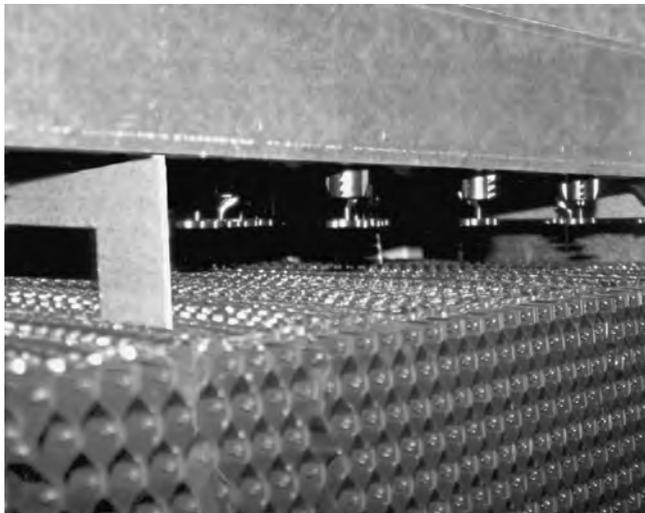
Eliminator air-seal removed showing nozzle distribution area above fill
